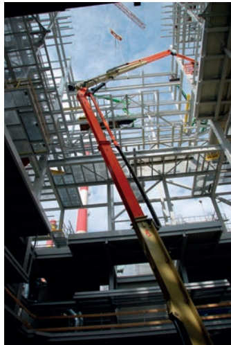
Fot. arch. Mostostal Kraków
