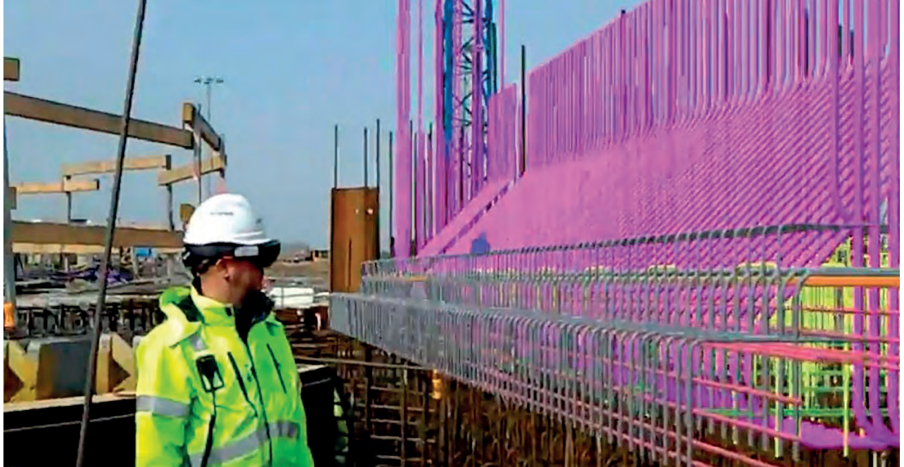
Fig.1. Visualization of the planned scope of works at the construction site with the use of augmented reality: European Spallation Source project in Sweden. Skanska materials, 2017
