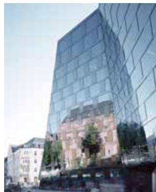
University Library Freiburg, Germany DEGELo ARCHITEKTEN www.degelo.net Photo © Barbara Bühler
