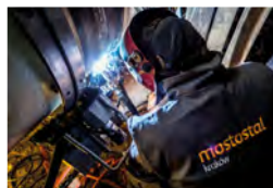
Fot. arch. Mostostal Kraków
