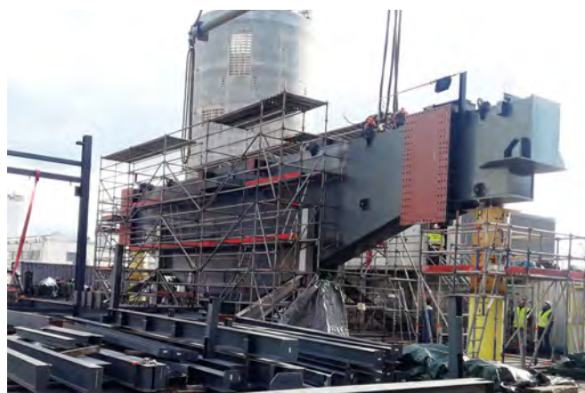
Fot. arch. Mostostal Kraków
