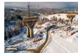
Fot. arch. ULMA Construction Polska
