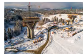
Fot. arch. ULMA Construction Polska
