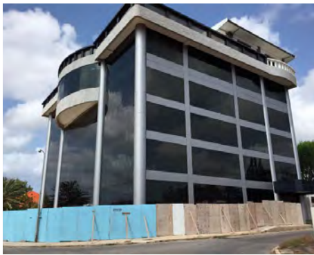
Fig. 6. Building to be investigated, Curacao 2014
